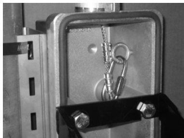
Lowering cable from the camera is attached to the eyebolt in the security lock box at the base.
